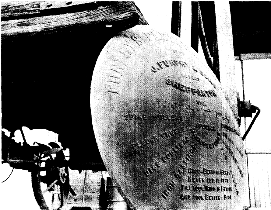
The cast end of the Furphy water-cart.
